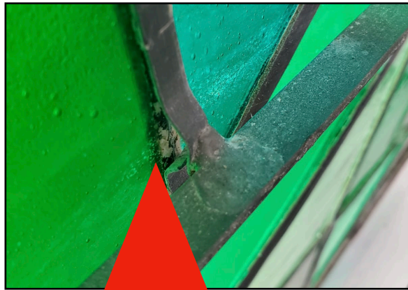
Stained glass is separating from the lead caming, causing glass to sag and loosen. This effects the overall structural integrity of the stained glass windows.
